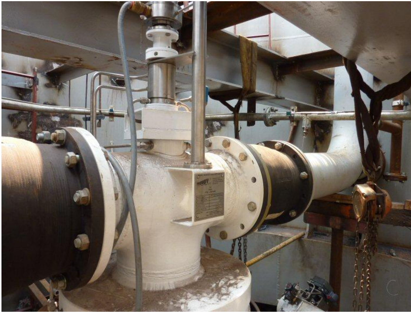
Swivel installed with 2 × 8" expansion pieces inside Turret Head
