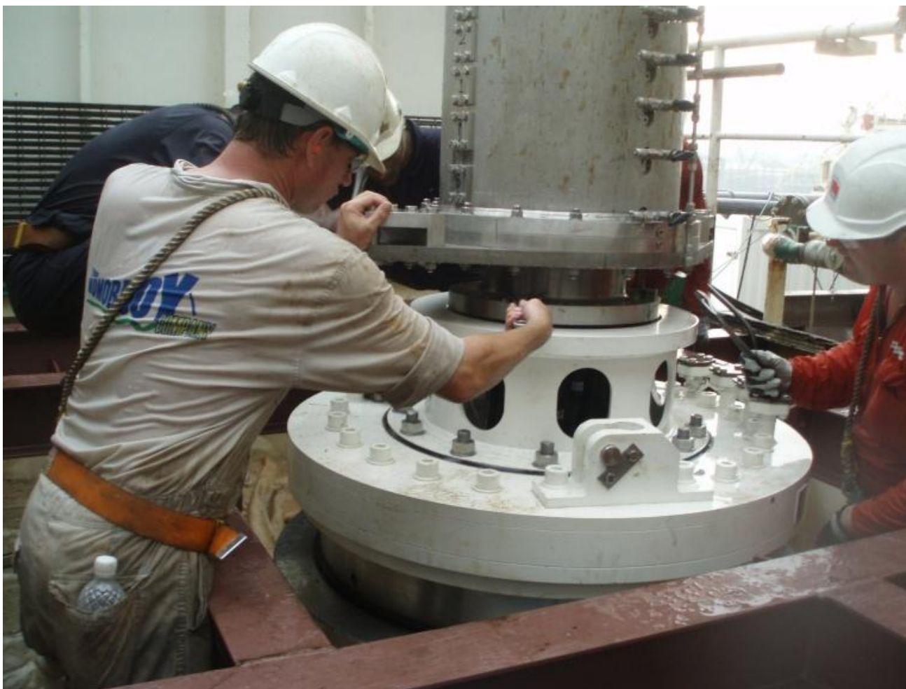
Swivel installation at Keppel
